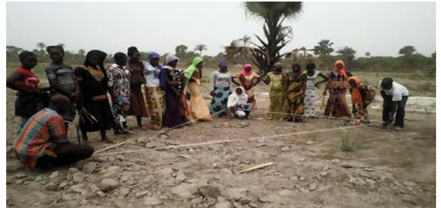
Demarcation using 3 - 4 - 5 method
